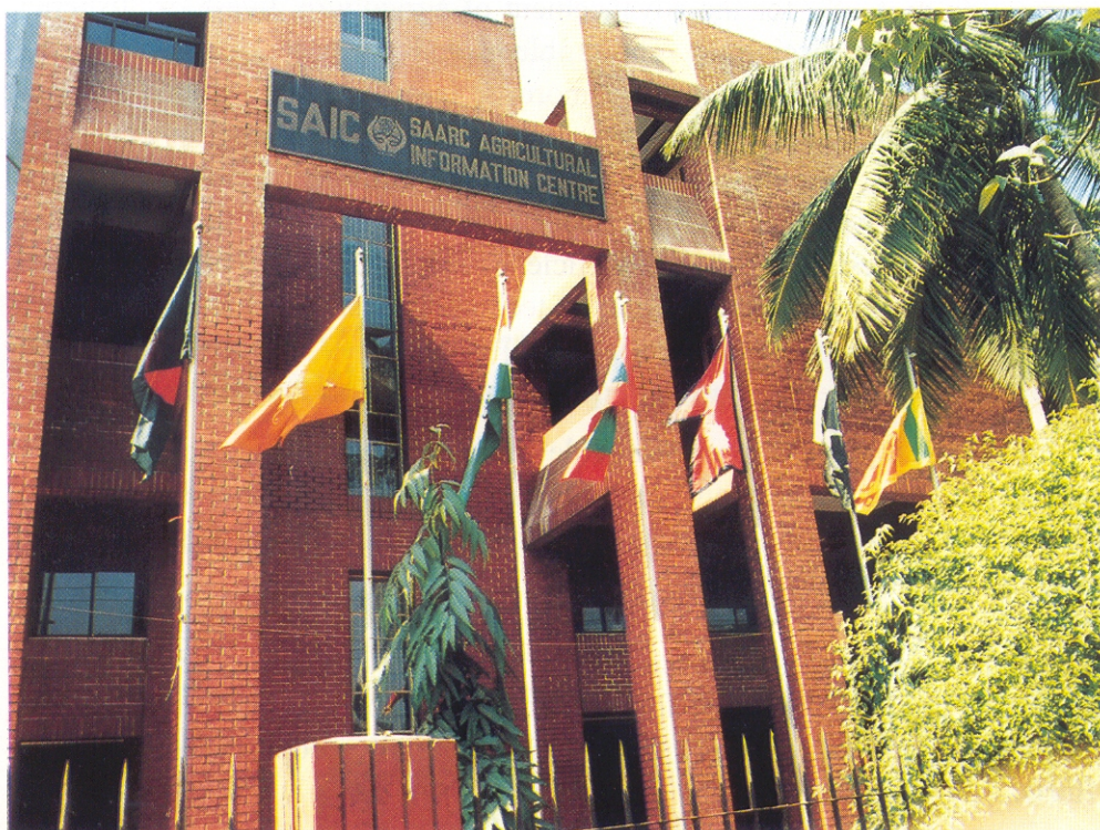
SAIC is housed in AIC Building of BARC
